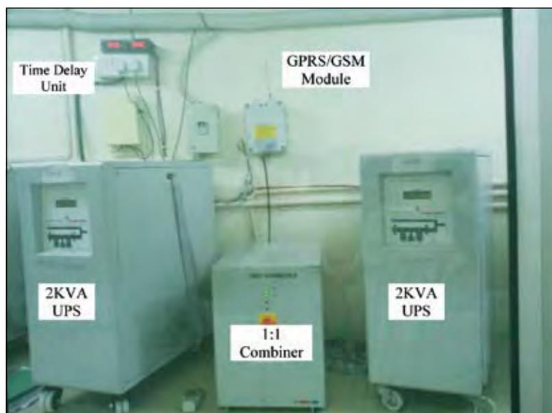
Fig. 4.19 One section of UPS room power packup with sms alert system
