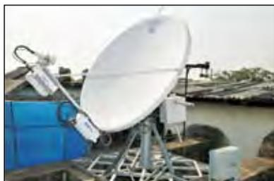
Fig. 4.11 Antenna unit of TWSTFT system installed on terrace of main building of NPL
