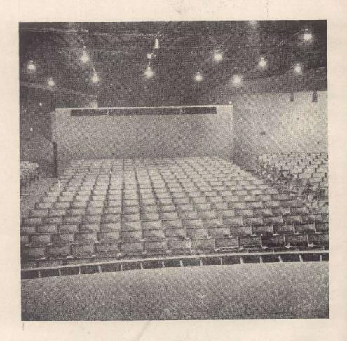
Fig. 6. Inside view of the Tagore Theatre Chandigarh from stage showing raked seats, resonators in back partition and exposed trusses in the ceiling.
