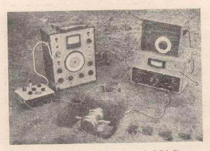
Fig. 4. Sound Attenuation Measurement in Soil in Situ. (a) Oscillator, (b) Amplifier, (c) Vibrator, (d) Pick-up, (e) Frequency Analyser, (f) Vibration pick-up preamplifier.
